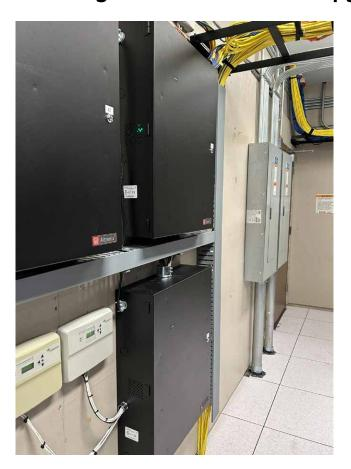
Unlike traditional access control systems that required large footprints, custom builds, or extensive rewiring, Altronix Trove2 access and power kits provide Cherokee Nation Entertainment with a compact, standardized solution. Each enclosure supported up to 16-doors within a small, manageable space—ideal for retrofitting existing casinos and facilities where space is at a premium.
